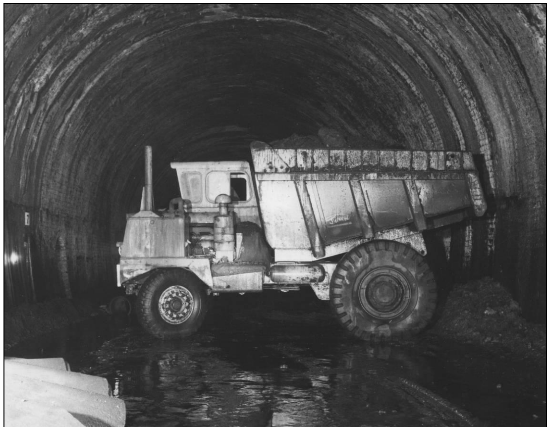
Fig. 6 The SL Dumptruck manoeuvring to approach the tipping area.
